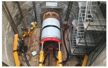
Once the Belgian contractor K-Boringen got awarded with the execution, the long-distance drive decided to throw many challenges at them such as extremely tight curve radii in alternating directions, sticky geology in combination with high and low overburden, high skin friction which resulted in high jacking forces, and many more...
