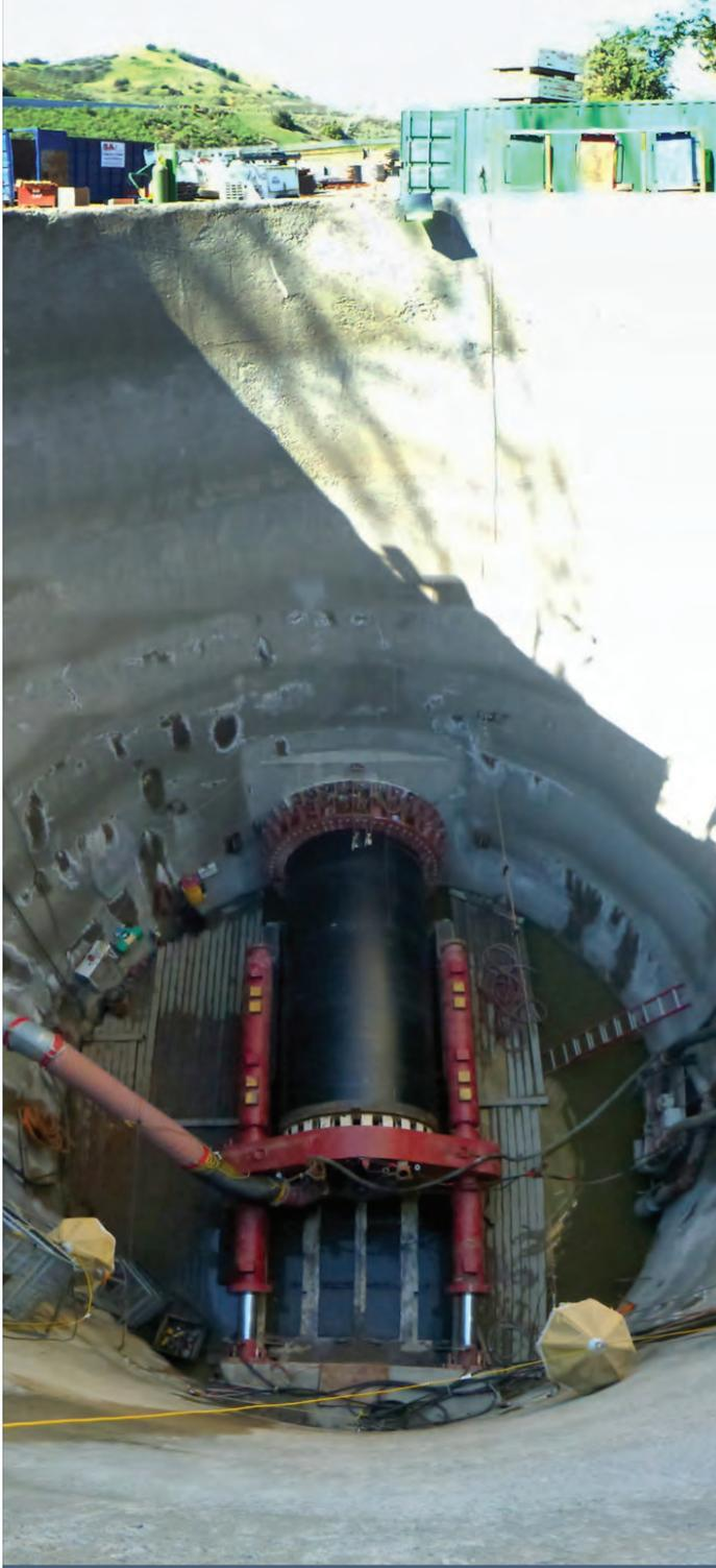
**PRIOR TO CONSTRUCTION, THE CONSTRUCTION TEAM PROPOSED COMBINING MULTIPLE DRIVES INTO A SINGLE, LONG S-CURVE DRIVE THAT WOULD ELIMINATE ONE SHAFT AND CONVERT ANOTHER TO A PUSH-THROUGH SHAFT.**
