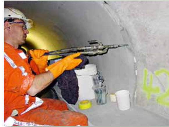
Carrying out sealing grouting
