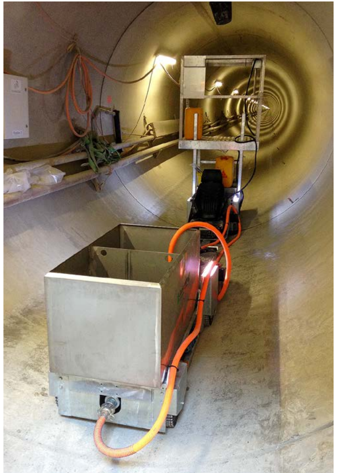
CT ROVER IN TUNNEL DN 3000 MM
