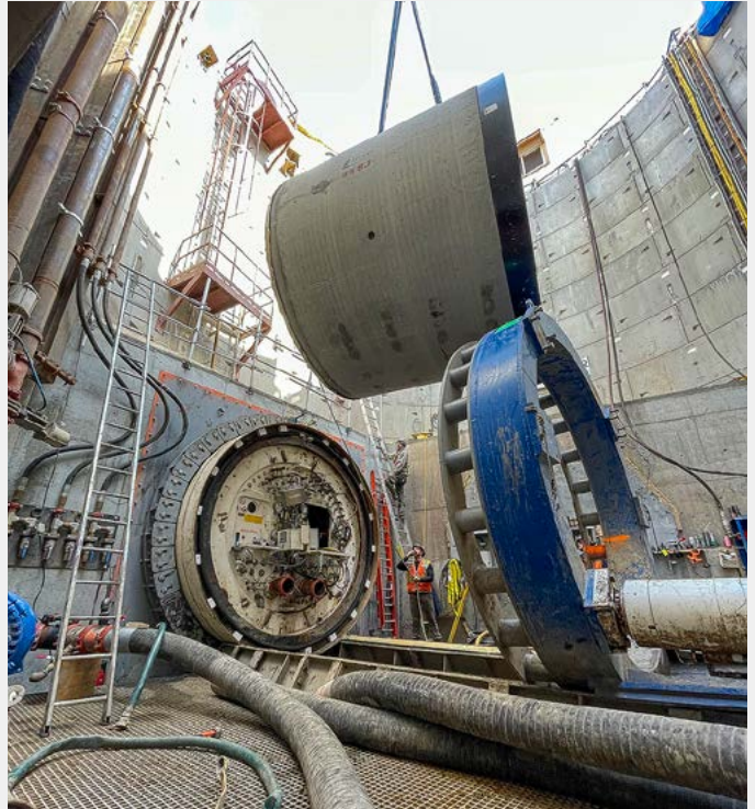
INSTALLATION FIRST PIPE IN STARTSHAFT
