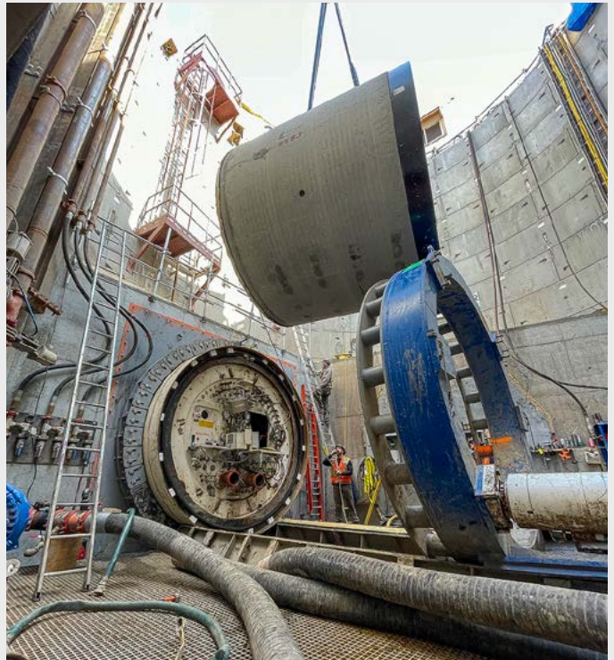
INSTALLATION FIRST PIPE IN STARTSHAFT
