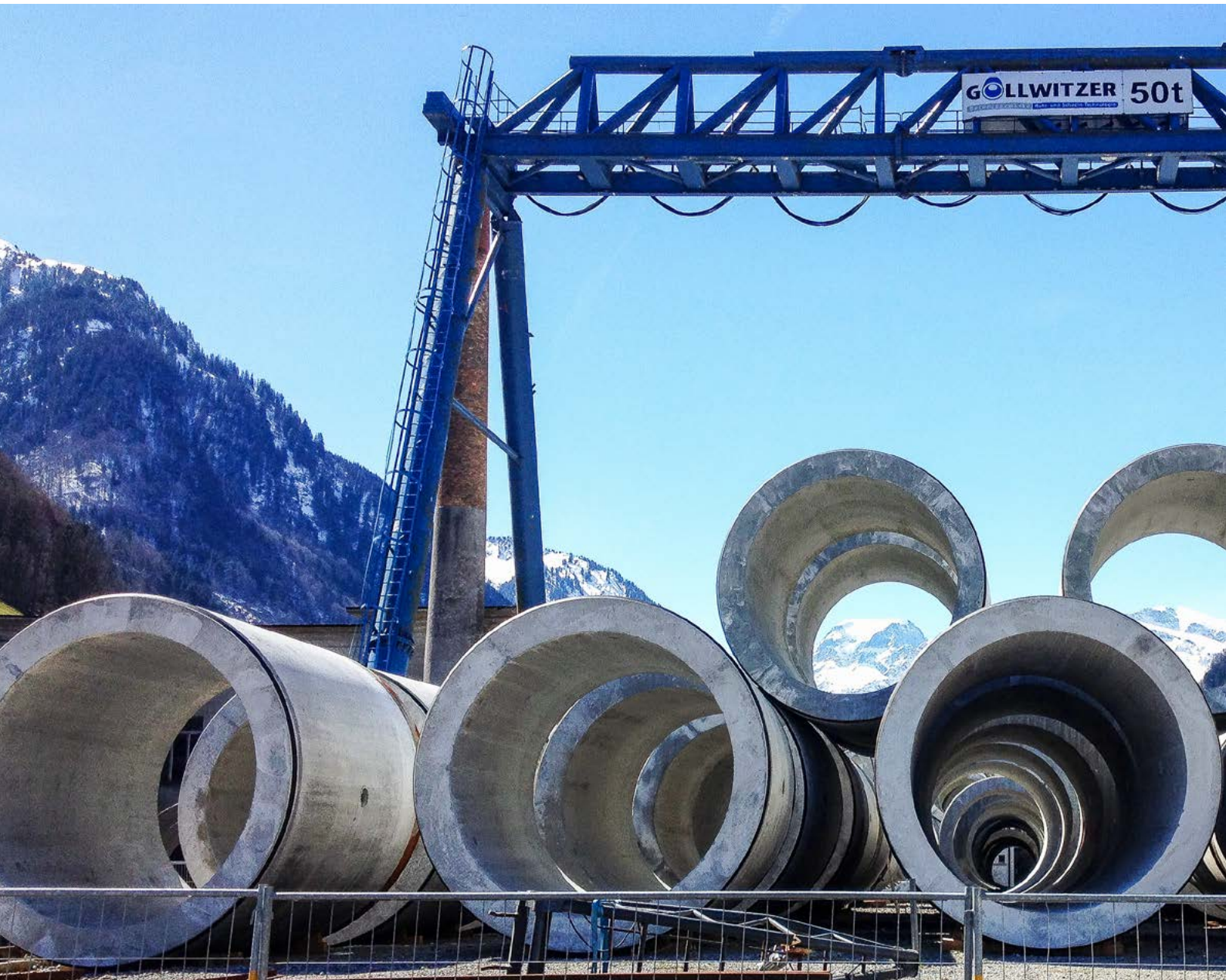
FIELD FACTORY FOR JACKING PIPES, SWITZERLAND
