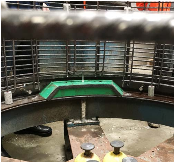
CAVITY FORMWORK ON PIPE SOCKET
