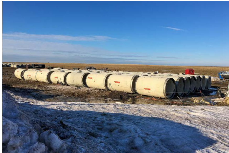
JACKING PIPES NORTH DAKOTA (USA)
