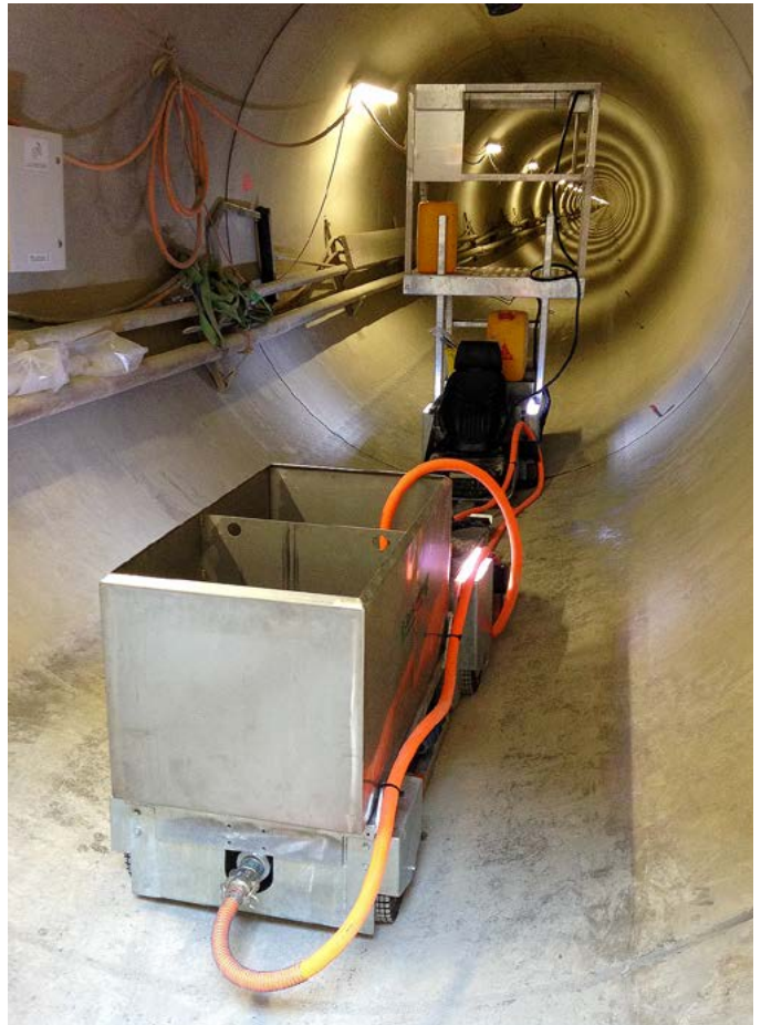
CT ROVER IN TUNNEL DN 3000 MM
