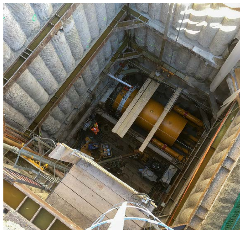
LAUNCH SHAFT IN SECANT PILE WALL
