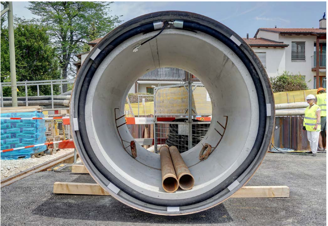
HYDRAULIC JOINT INSTALLED ON A REINFORCED CONCRETE JACKING PIPE
