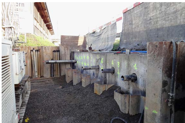
PIPE ROOF, SWITZERLAND
