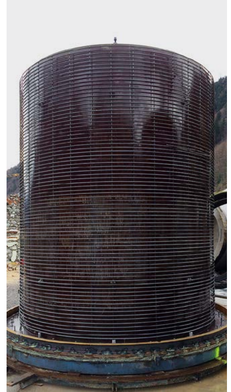
REINFORCEMENT CAGE OF RC PIPE IN MOULD
