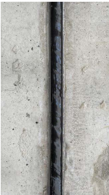
VIEW OF CAVITY AREA FOR HYDRAULIC JOINT TREATED WITH JCFlex
