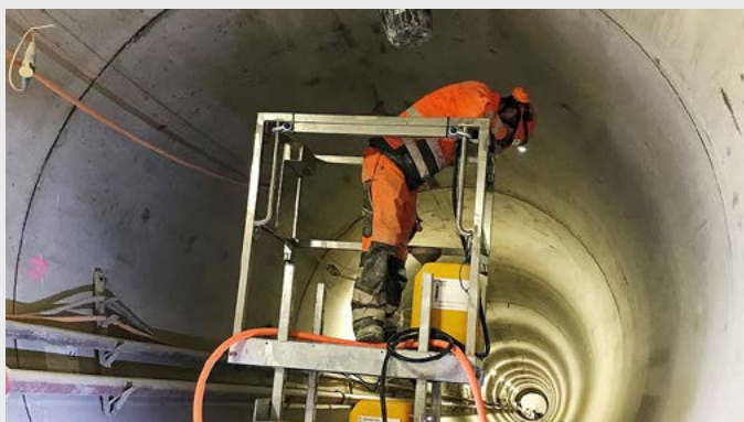
JCGrout CEMENT PASTE INJECTION: CTROVER IN THE TUNNEL FOR GROUTING WORKS
